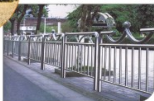
室外护栏 Outdoor guard rail
