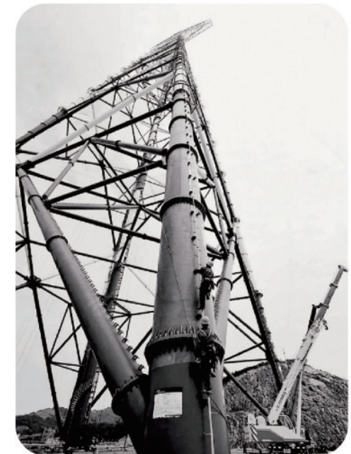
钢管塔 Steel pipe tower
