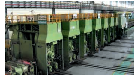
精轧机 Finishing mill
