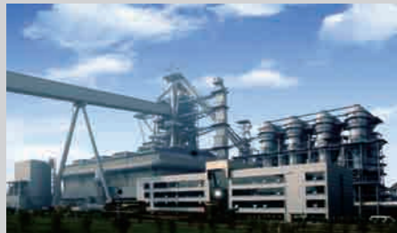
4350高炉 4350 blast furnace
