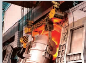
180吨顶底复吹转炉 180 ton top and bottom combined blown converter
