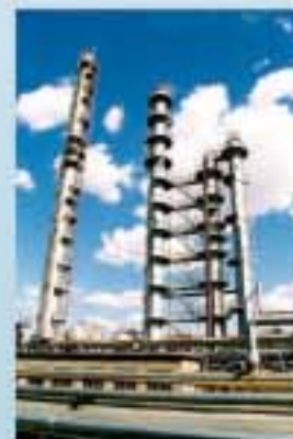
石化厂 Petrochemical facility
