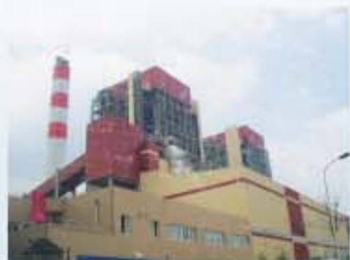
电站锅炉 Power station boiler
