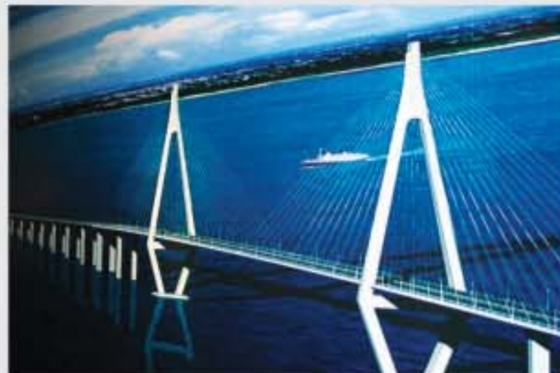
杭州湾跨海大桥 Hangzhou Bay Cross-sea Bridge
