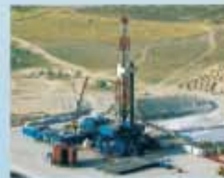
陆地石油钻井 Inland oil drilling
