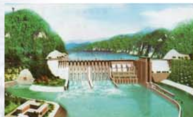
向家坝水电站 Xiangjiaba Hydropower Station
