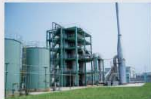
垃圾焚烧厂 Waste calcinations plant
