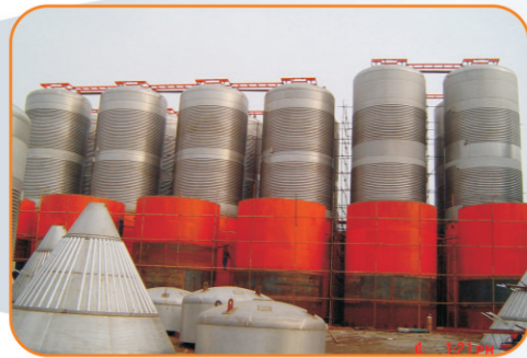
储罐 Storage tank
