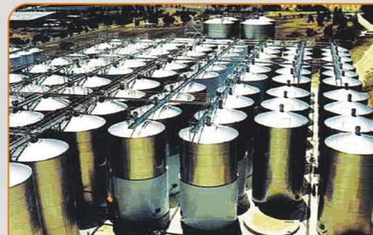
酿酒加工罐 Brewery tank
